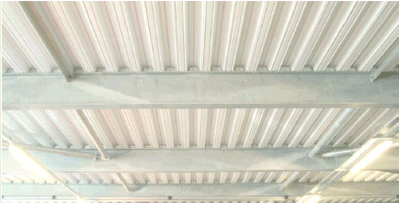
STEP IN DECK FLOOR
